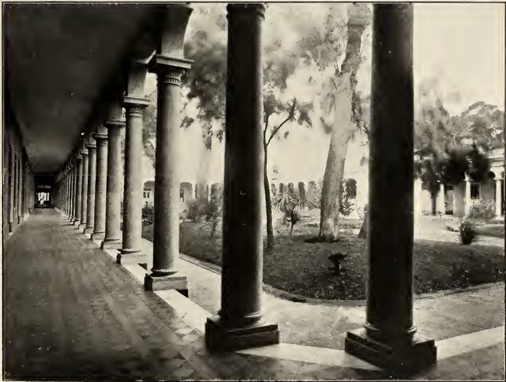
CORRIDOR AND COURTYARD OF THE SAN ROQUE HOSPITAL.
